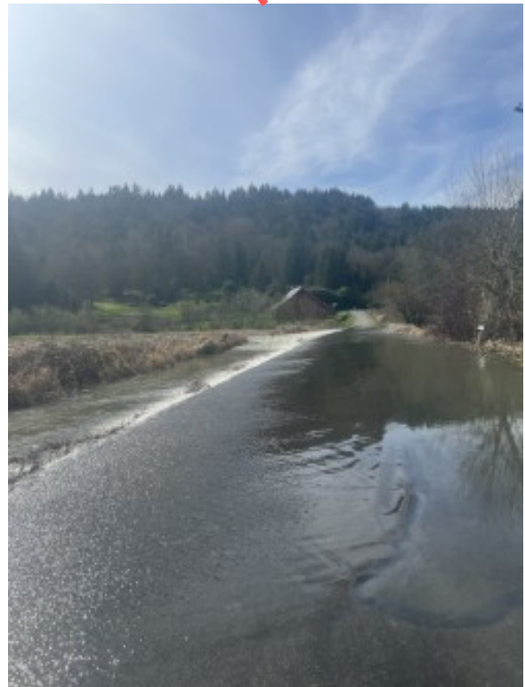
3:13pm, headed west towards Goose and Gander farm along 100 th St. Water still spilling over road from north fields into southern fields where gauge is.
